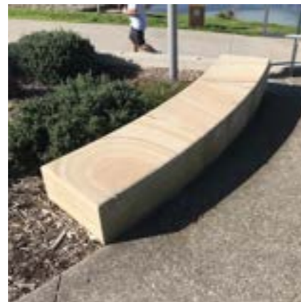
Curved sandstone plinth walling
