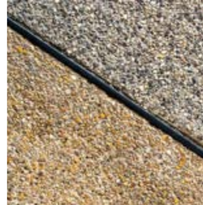
Exposed aggregate-jointing
