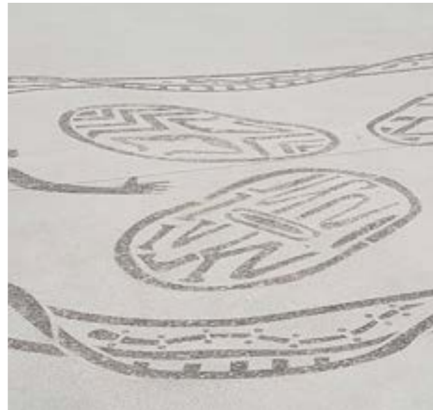
Exposed aggregate-Pavement Art
