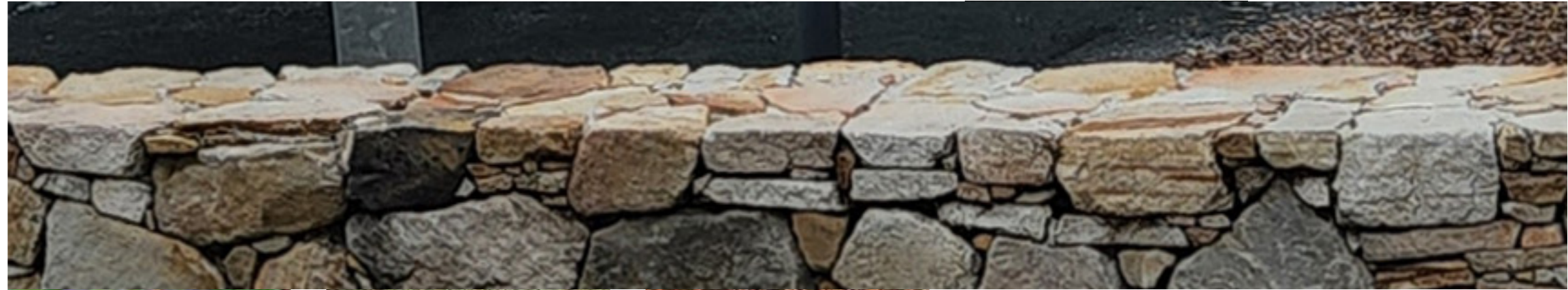
Sandstone walling to match existing at Riverside Park
