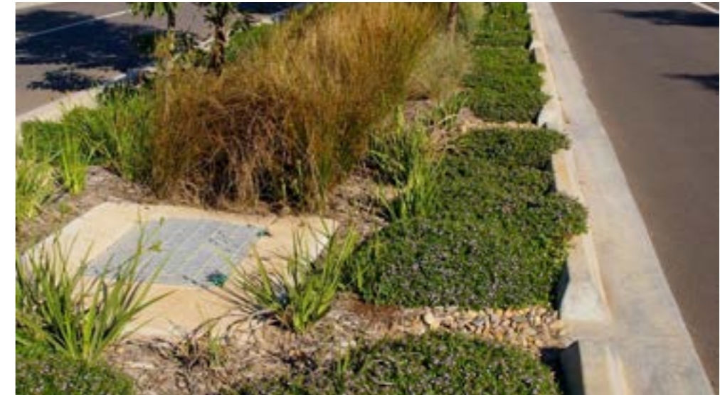
Passivley watered gardens-Kerb inlets
