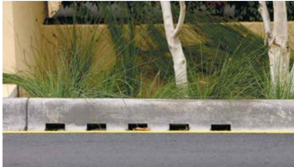
Passivley watered gardens-kerb inlets
