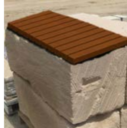
Wooden slat bench seating to stone walling
