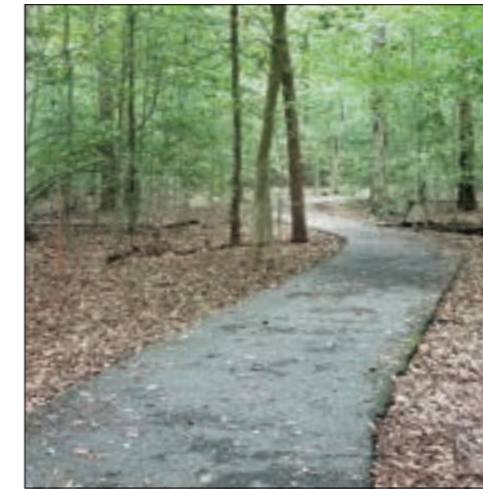
Figure 35: 2000mm asphalt pavement.
