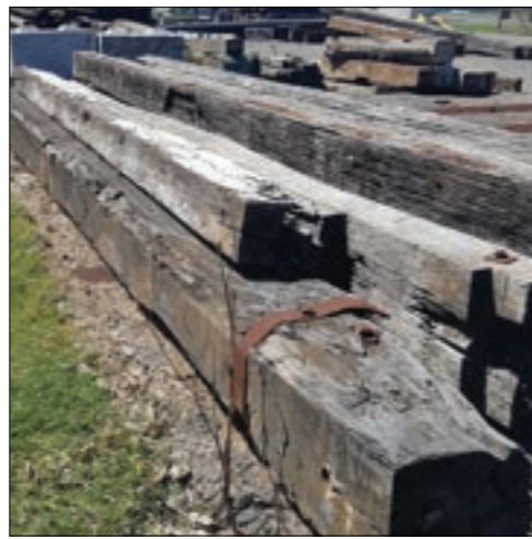
Figure 46: Local recycled bridge timbers to detail crossings.
