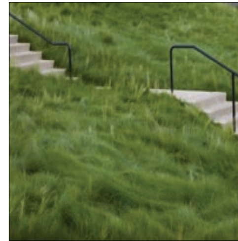
Figure 36: 2000mm concrete stairs.
