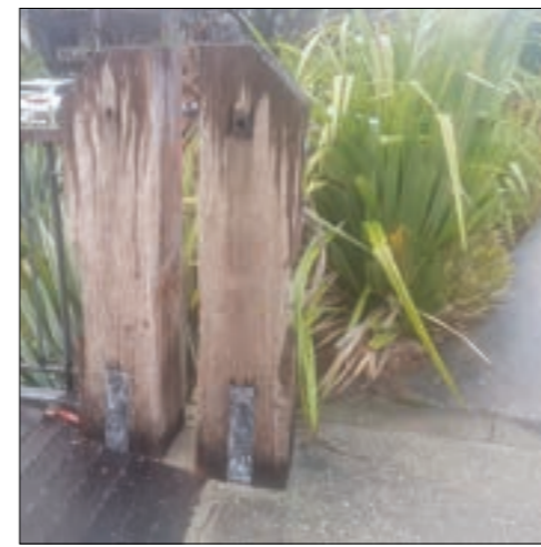
Figure 47: Example of bridge detailing.
