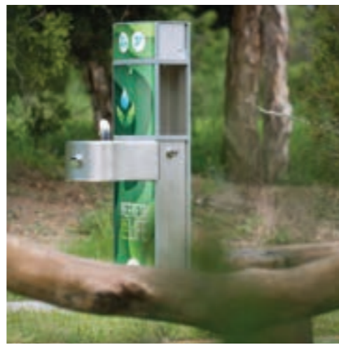
Figure 20: Water refill and drinking station.
