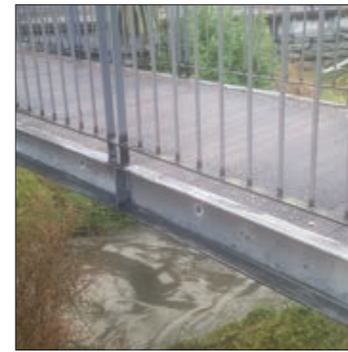
Figure 48: Example bridge crossing balustrade.
